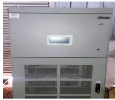
After- 3 level IGBT based Static Var Generator (SVG) with inverter based technology to reduce delta between kVAh & kWh achieving power factor up to 0.999. Compensation with less than 15 milli second response time. 200 KVAR. Now PF is 0.999
