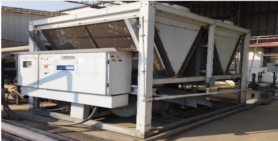
Before- We used 75 TR air cooled chiller, consuming 78 unit/hr. at 100% loading & its \text{kWh/Tr} is 1.04
