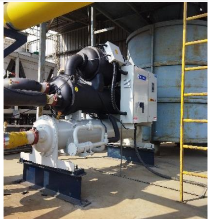
After- Replaced with 125TR water cooled chiller, consuming 45 unit/hr. at 58 to 60% loading. & its \text{kWh/Tr} is 0.49
