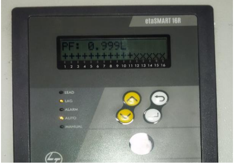
After- 3 level IGBT based Static Var Generator (SVG) with inverter based technology to reduce delta between kVAh & kWh achieving power factor up to 0.999. Compensation with less than 15 milli second response time. 200 KVAR. Now PF is 0.999
